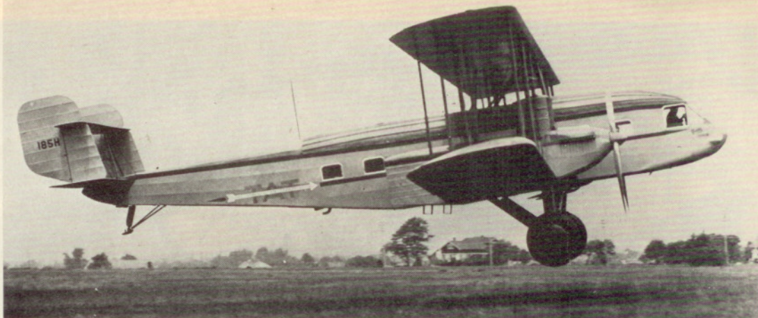
The first three Condor transports used the bomber wings, tail, and nacelles, but stretched the fuselage to accommodate a cabin for 18 passengers, two pilots, and a steward.
